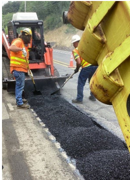
Asphalt Repairs
