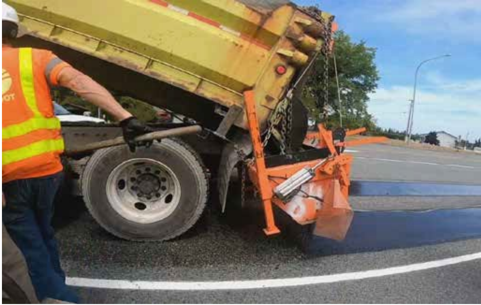
Figure 4-1: Wheel-path Chip Sealing
