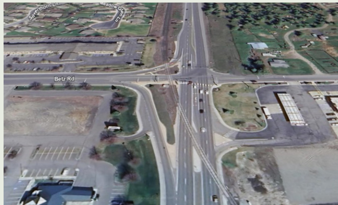
Betz Road and State Route 904 with rail crossing
