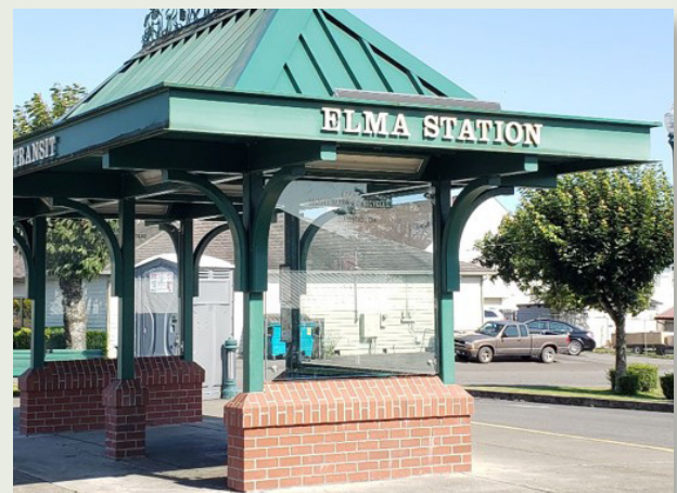
Grays Harbor Transit Station, Elma, WA
