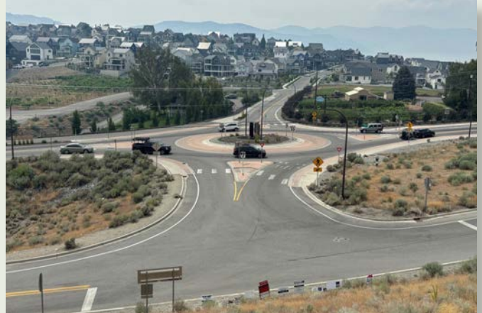
State Route 150 Roundabout serving Chelan County
